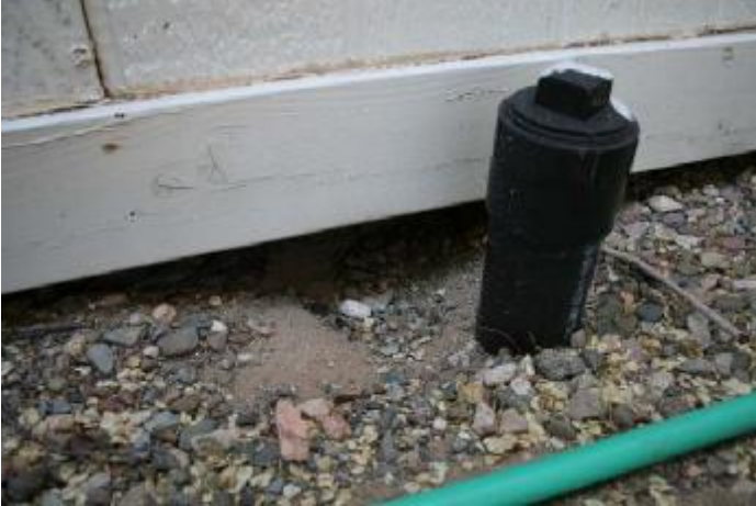
1. The soil slopes towards the house in the front. Regrade the soil around the foundation so
